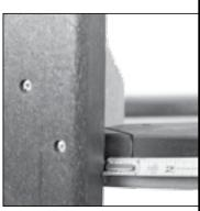
Align boards so they run the same direction as the boards in the tabletop. Position the side of the legs 3/4" from the nearest joint in the shelf boards. Fasten each brace to the shelf with a 21/2" screw. Then fasten the legs to the shelf with two 21/2" screws in each leg using the pilot holes in the legs.
